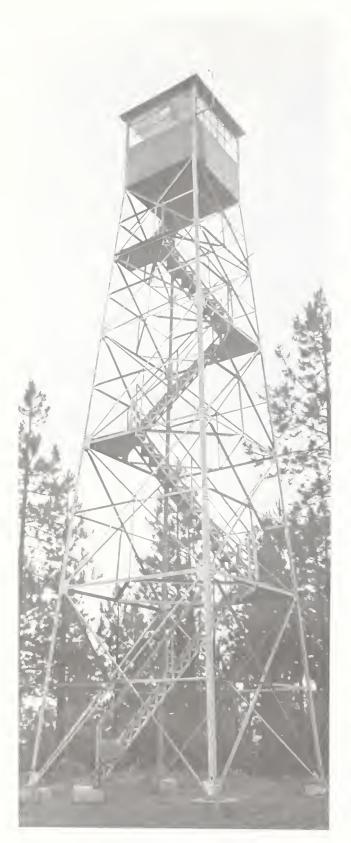
Figure 75. PS Knoll lookout built by the CCC in 1939 on the Apache-Sitgreaves National Forests. This is an Aermotor MC-40 type and is 45 feet tall. The view is looking to the south east.
